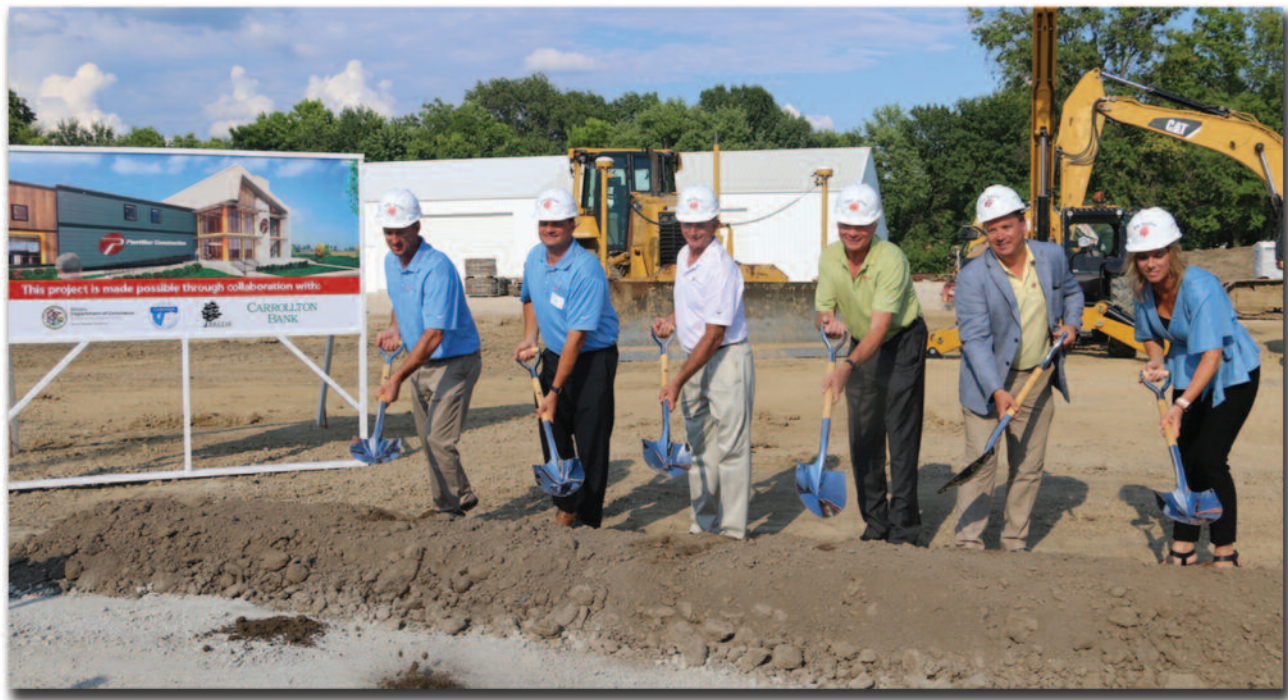
Poettker Construction Groundbreaking: A new 12,000 sq. ft., $30 million headquarters is being built in Breese. The project should be complete in late 2019.
